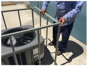
**Step Five:** Slide in the service access panel and secure the panel with four #10 x 3/4 self-drilling screws on both sides, top and bottom.
