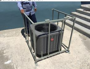
**Step Four:** After joining the first side panel to the long panel, repeat steps two/three to join the second side panel to the long panel and align the cage over the condensing unit.
