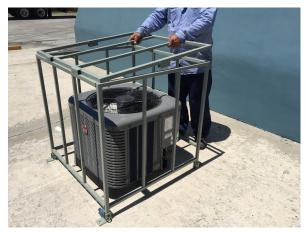
**Step Six:** Insert the top panel by sliding it into the long panel's holding brackets, and insert the longer padlock through the top panel's hole to secure the condensing unit. The cage is now ready to be anchored.
