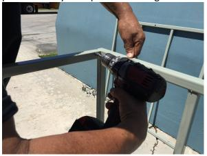
**Step Three:** After joining one of the side panels into the long panel, ensure that both holes on top and bottom are aligned and insert two #10 x 3/4 self-drilling screws.
