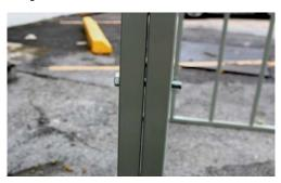
3. Insert the 3/8"x2 1/2" bolt into the aligned holes between the hinged dual panel and single long panel.
