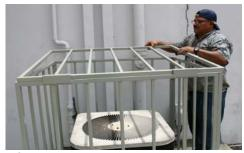
7. Slide the top panel under the angles. Line up the predrilled holes opposite the angles.
