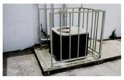
4. Position the cage around the condensing unit.
