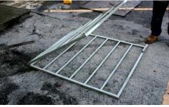
2. Open and stand the hinged dual panel on the pre-installed swivel feet
