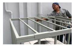
8. Install padlock in predrilled holes opposite the angles to secure cage. SQUARE THE CAGE, and anchor to the pad (anchors not supplied).
